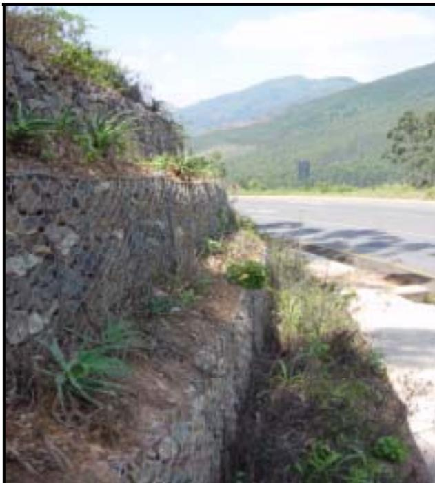
The placing of topsoil and the planting of Aloes and other selected plants have resulted in an aesthetically pleasing vegetation cover along the full extent of the gabion walls.
