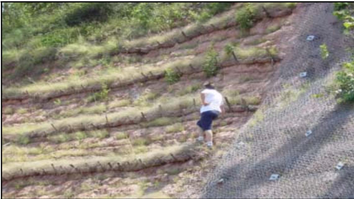
The hydroseeded grasses between the rows of vegetation cylinders or compost rolls and vetiver grass hedge rows have established in the horizontally "scarified" or "ridged" rows.
