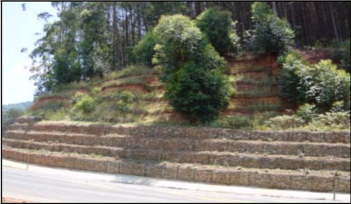
The view of the protected side slope demonstrating the combined use of gabion walls and the erosion control methods deployed have successfully achieved the required stability. Little or no silt deposits can be observed along the full extent of the concrete side drains.
