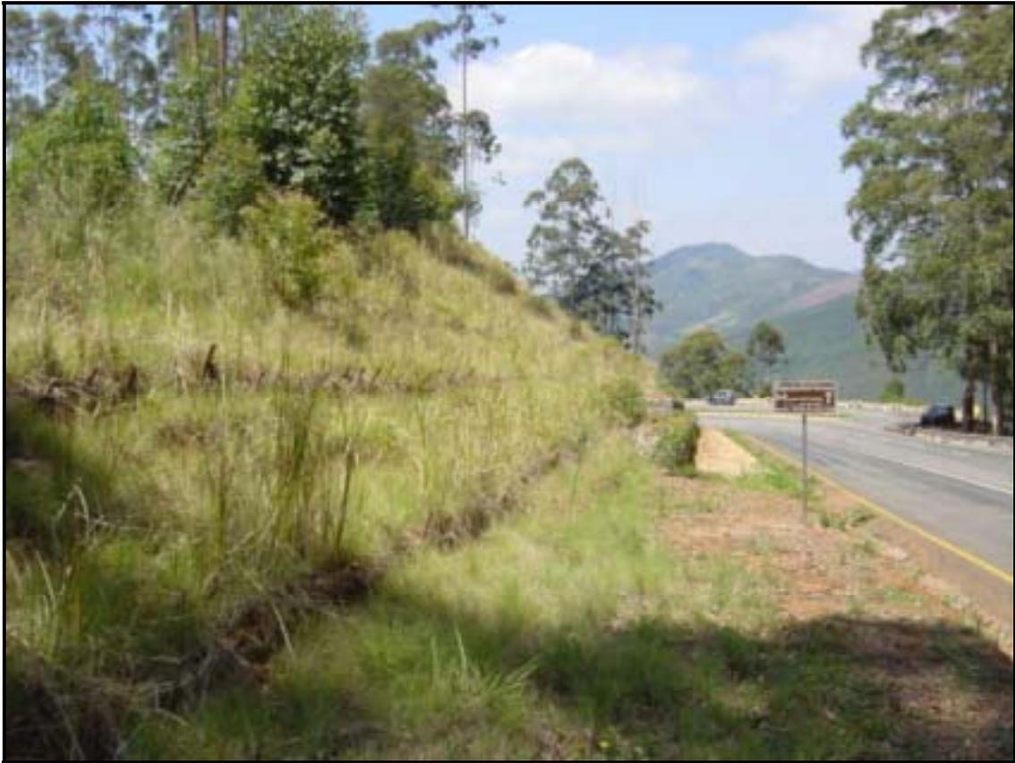
The combination of the installed rows of vegetation cylinders or compost rolls, planted vetiver grass hedge rows, application of selected grass seeds incorporated into the hydroseeding mixture and with the gabion baskets has resulted in a stable environmentally acceptable vegetation cover being attained.
