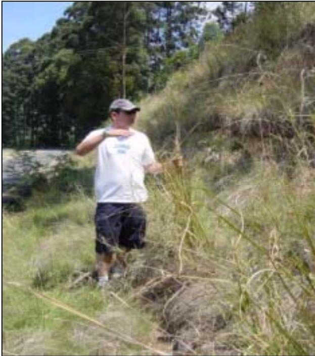
The Vetiver grass hedges have established well behind the rows of vegetation cylinders or compost rolls. The average height of the plants vary around 1200mm in the more fertile soils and around 450 mm along the steep slope areas where little soil is present. The various grass species incorporated into the hydroseeding mixture is clearly visible along the full, extent of the scarified side slope and is well developed.
